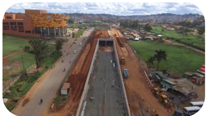
Aerial View of the Underpass (Mukwano Side)
