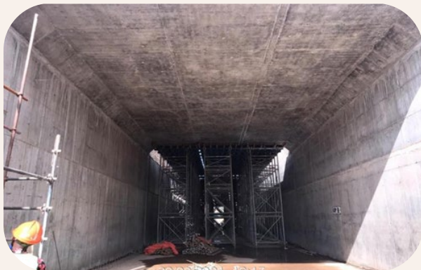
Finished F3 Surfaces of the Underpass Walls and Top Slabs
