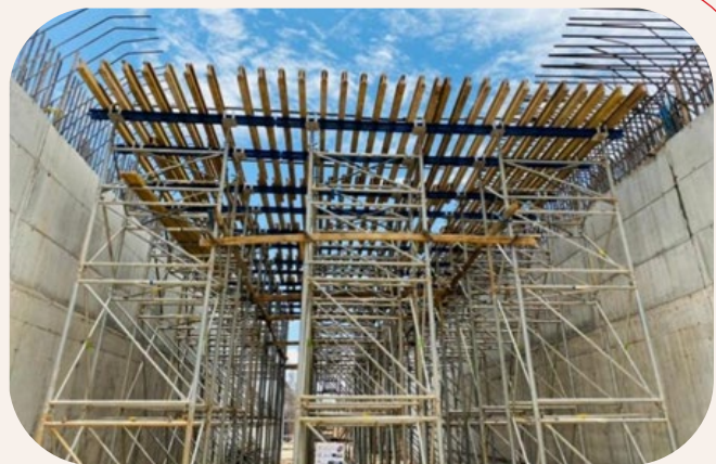
Top Slab Formwork Set Up using DOKA D2 Towers (Load Capacity of 57.6kN per Leg)
