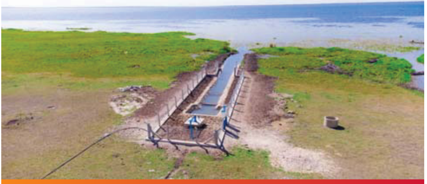
Figure 1. Completed Agule intake structure of channel, silt basin and sump
